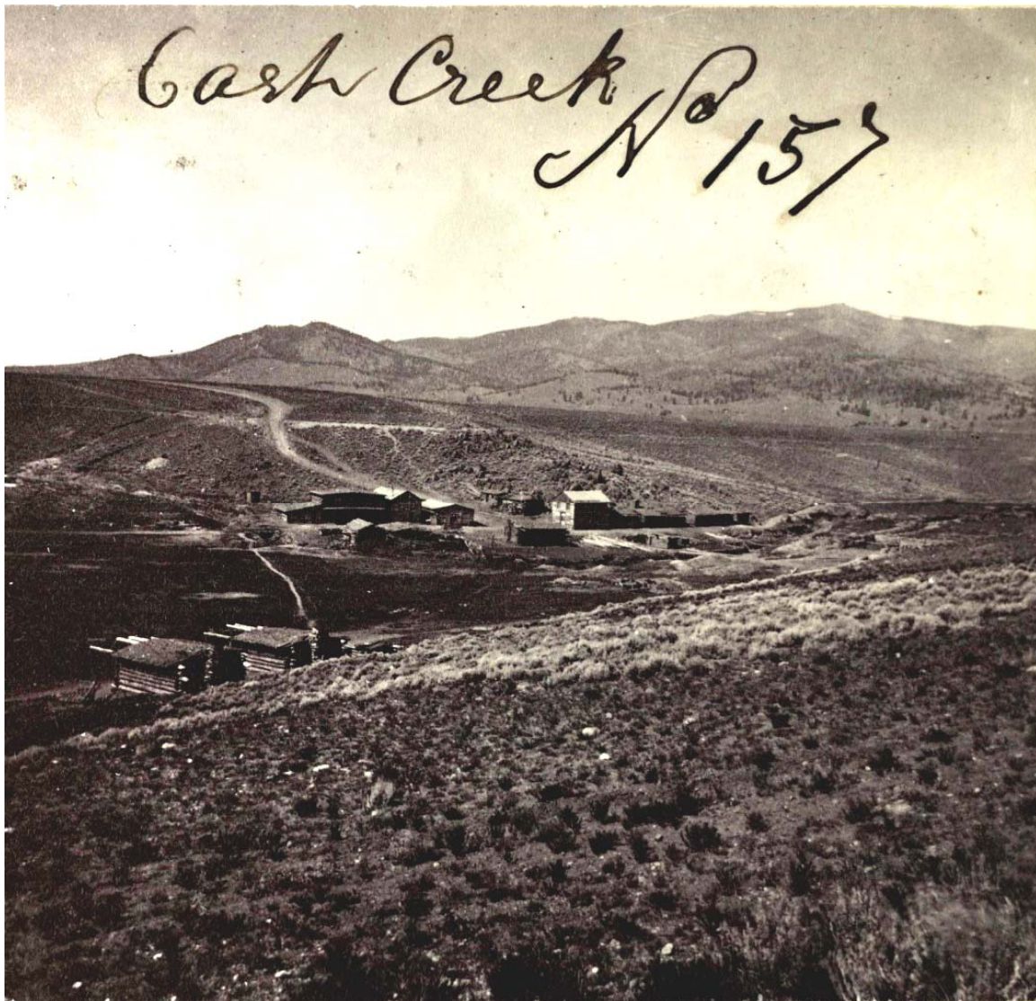
FIGURE 1. View of cabins and buildings in Cache (Cash) Creek (Park County, later Chaffee County), Colorado. The Cache Creek ditch, stretching 16 miles from Cache Creek Park to Lake Creek, was completed in 1863 and brought water to the goldfields for mining operations. Photo date is between 1865 and 1875 by William G. Chamberlain. Source: from a "scrap" book of Denver and Colorado of William G. Chamberlain, Photographer, 1861-1881. Courtesy of the Denver Public Library, Western History Collection, William G. Chamberlain, Call Number X-19192. © Denver Public Library.
