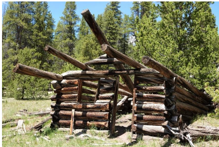
Figure 3. A Pieplant miner’s cabin along a meadow. The long poles supported a porch roof. Photo date 7/2020 by S. Veatch.
