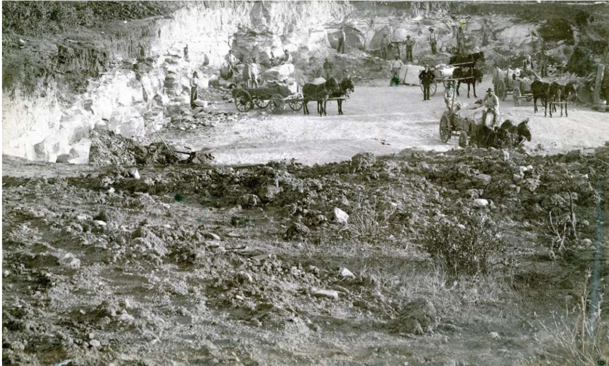
Figure 6. View of the Madge quarry, later known as the Douglas quarry. Wagons are loaded with blocks of rhyolite. Unknown photographer. Photo date circa 1890s. Courtesy Douglas County Libraries Archives & Local History, no. 1997.011.0678.0002.
