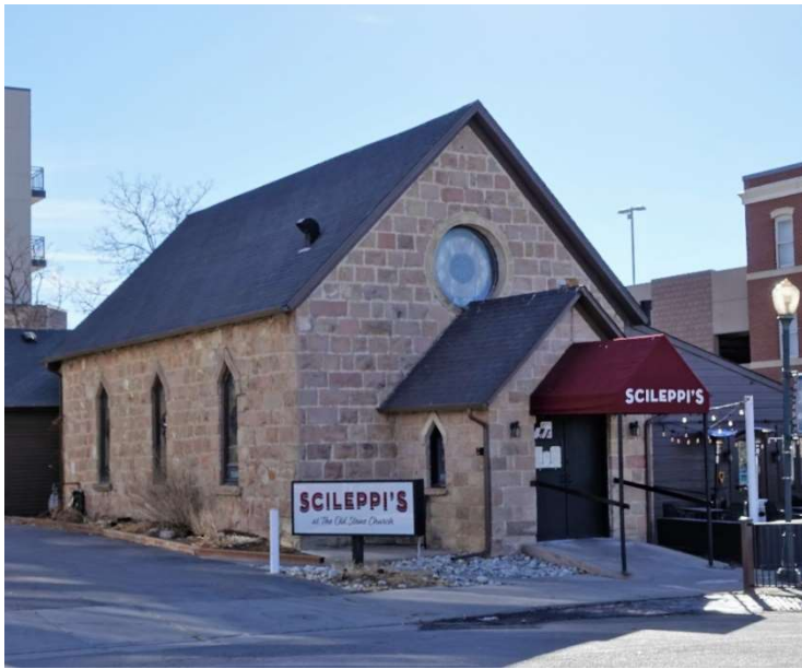
Figure 4. St. Francis of Assisi Catholic Church built in 1888 with rhyolite (now Scileppi's at the Old Stone Church Restaurant). Photo date 2021 by S. W. Veatch.
