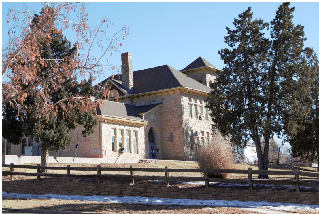
Figure 3. Cantril School built in 1896 with Castle Rock Rhyolite. Photo date 2021 by Ben Elick.
