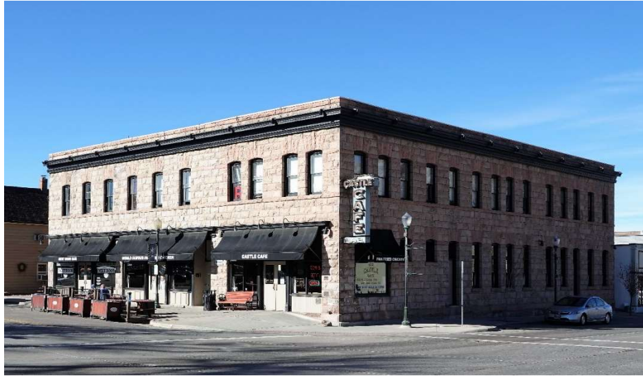
Figure 2. Castle Rock Café. Built with local rhyolite blocks. Photo date 2021 by S. W. Veatch.
