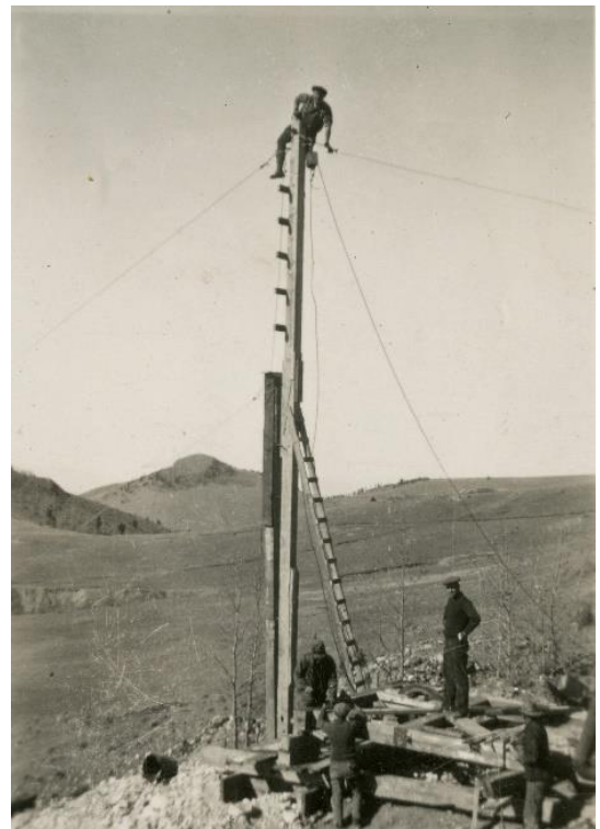
Figure 7 Sutton sits on top of the gin pole and attaches the guy wires to stabilize it. Photo date circa 1932. William Sutton collection, courtesy of the Cripple Creek District Museum.
